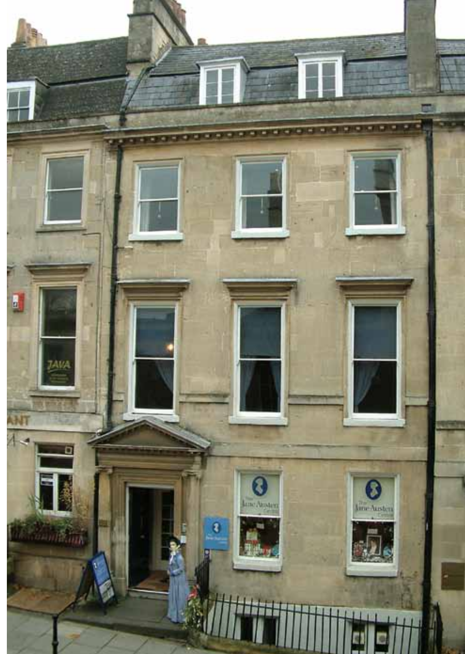
Jane, herself, lived very close to the Jane Austen Centre in 1805, higher up the hill at No. 25 Gay St. This and other landmarks can be seen on the Jane Austen city walking tour that meets daily at the KC Change Visitor Info Centre.
